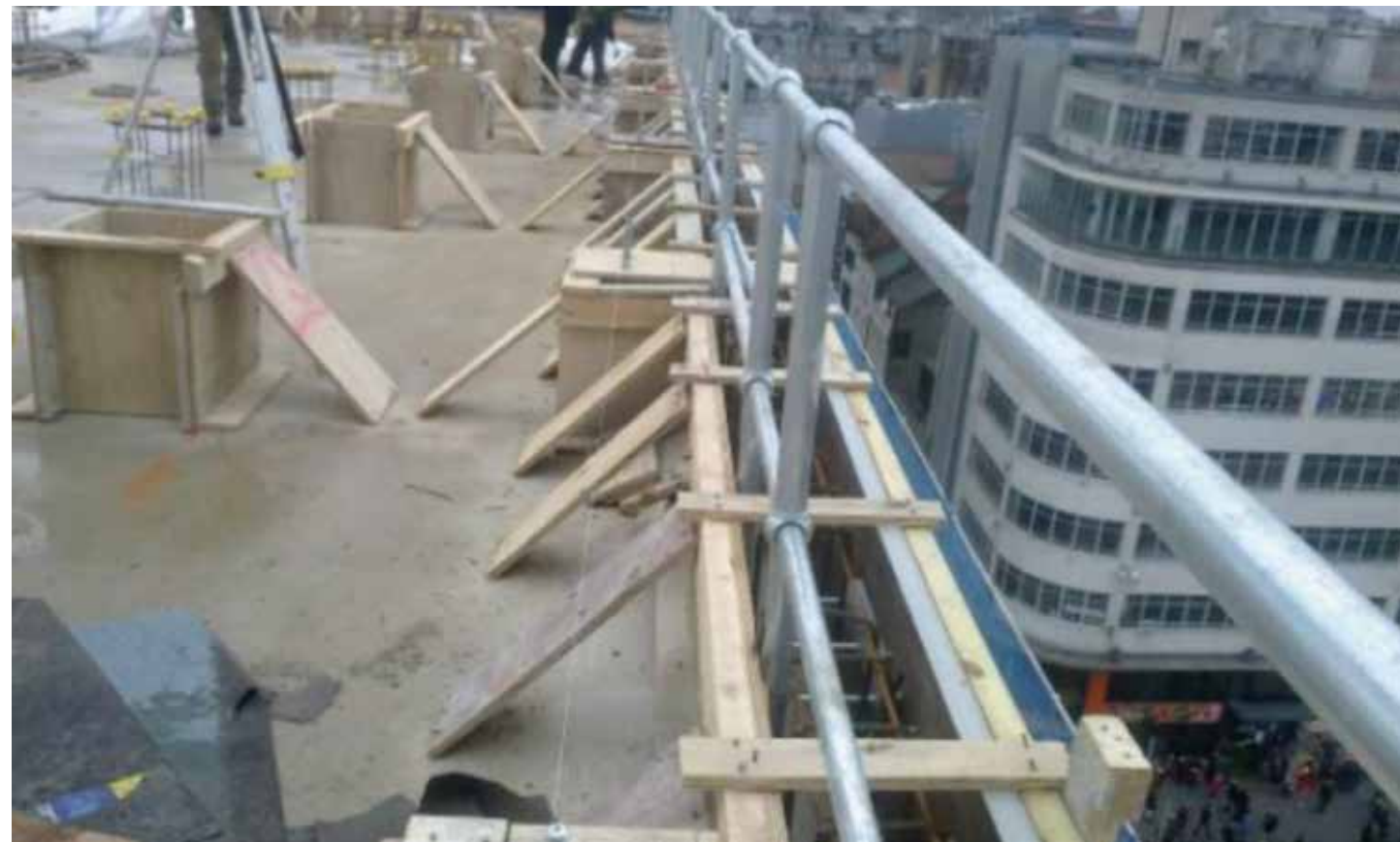
Alignment checked before pouring
