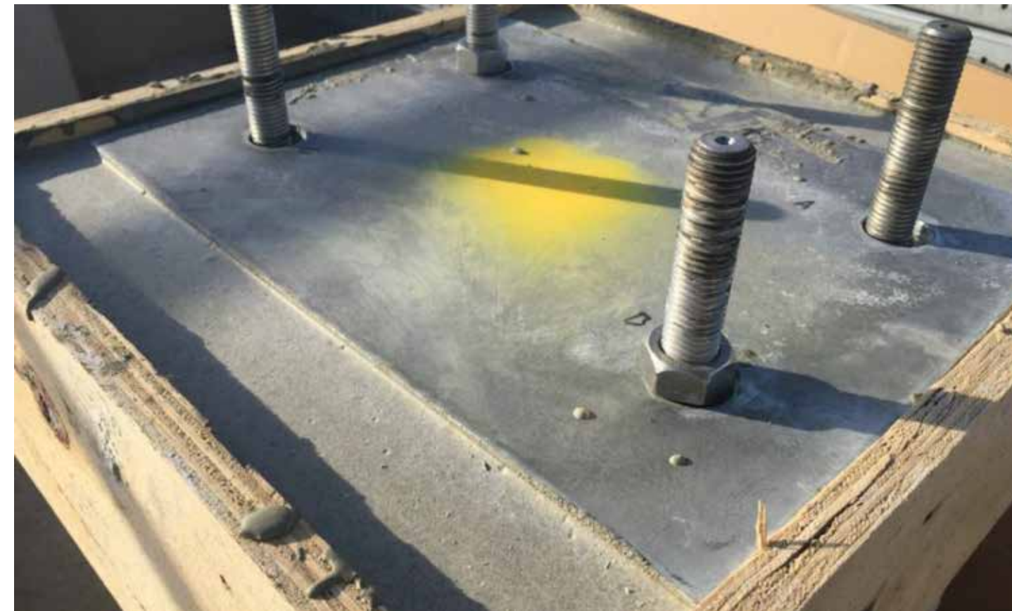
Bed plate installed and grouted in
