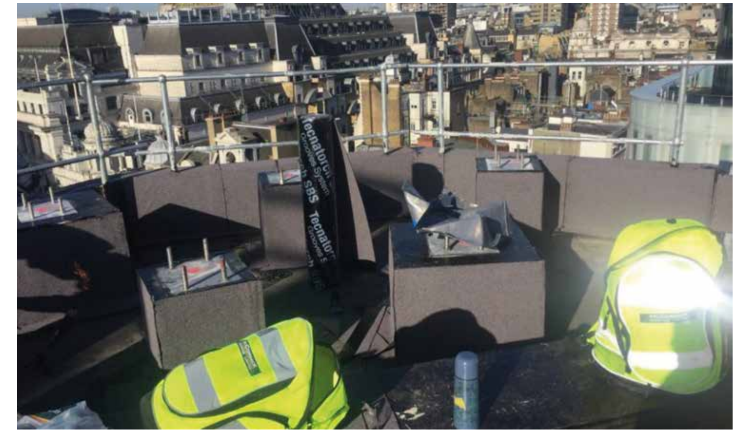
Insulation applied
