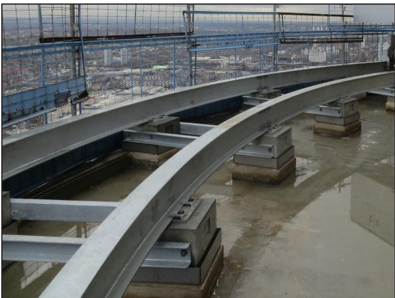
Complete installation of Hold Down Unit & Track
