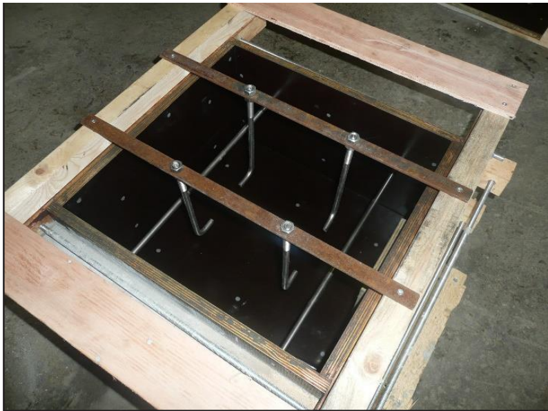
Pre-pour set up of HDUs & fixing bolts
